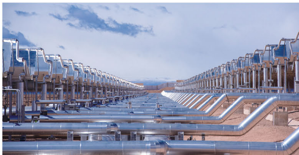
镜场导热油小管道保温工艺 Heat preservation technology of mirror field heat transfer pipe line
